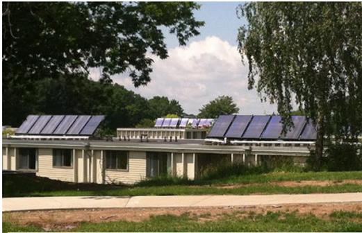
*Syracuse University installed 20 solar thermal panels on South Campus apartment buildings in 2013 to provide domestic hot water.*
