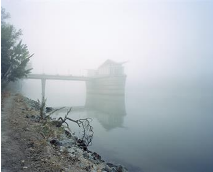
“Water Intake, Sacramento (2016)”
